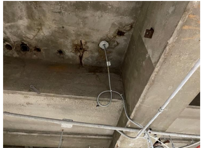
Photo LAUN-S1: Spalled Concrete at Floor Penetrations
