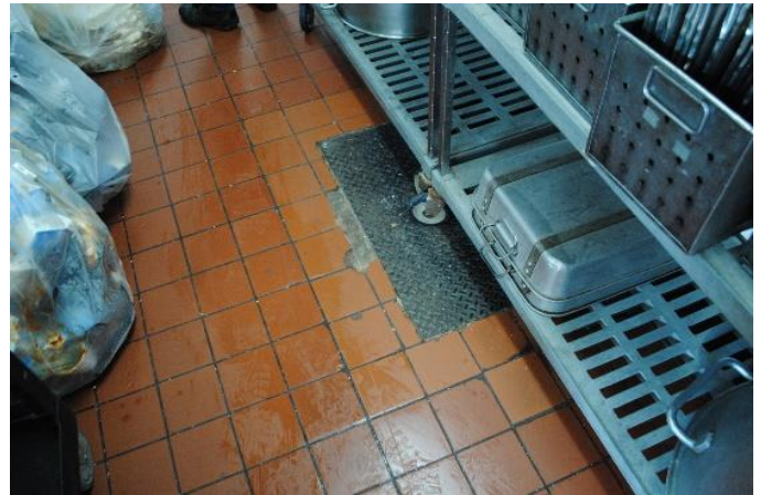
Photo HU6-A2: Floor Tile Damage and Missing in Kitchen
