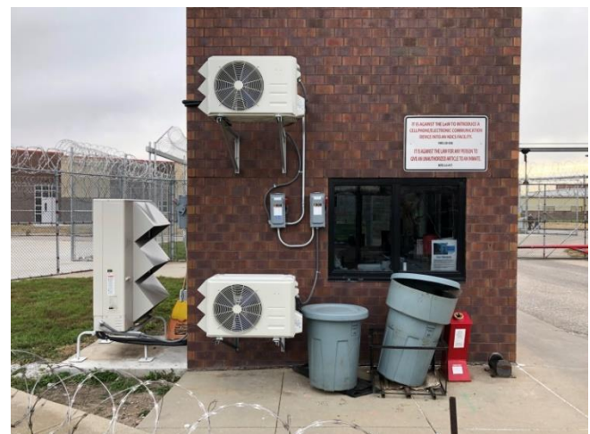
Photo GT2-M3: Existing Air-Source Heat Pump
