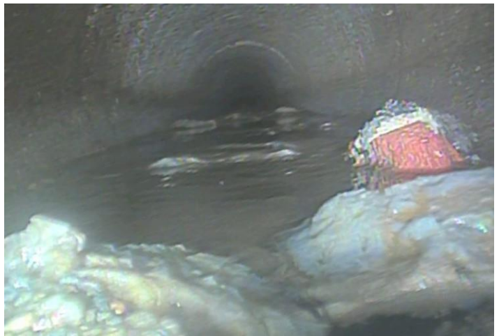
Photo SAN-1: Debris Found in SAN Piping
