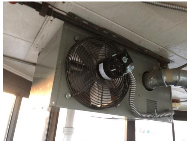
Photo GT4-M2: Existing Gas Unit Heater
