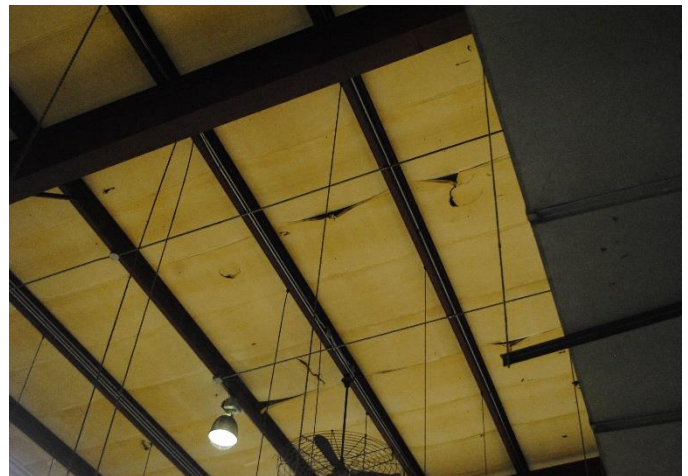
Photo PVB-A1: Tears in Insulation at Ceiling
