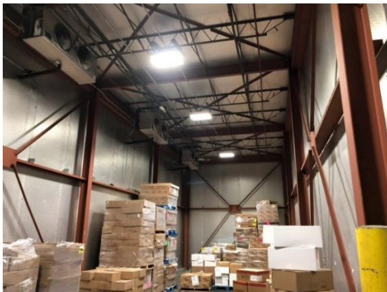
Photo CW-FS1: Existing Freezer Evaporator Coils
