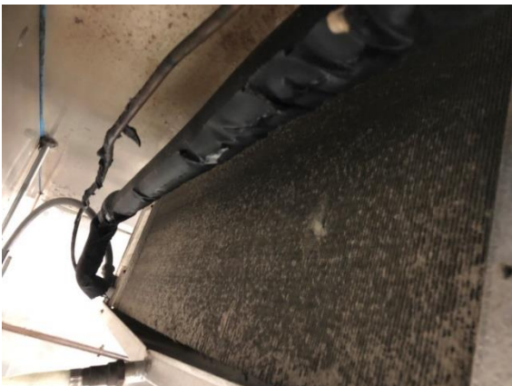
Photo HU6-FS3: Existing Cooler Evaporator Coil
