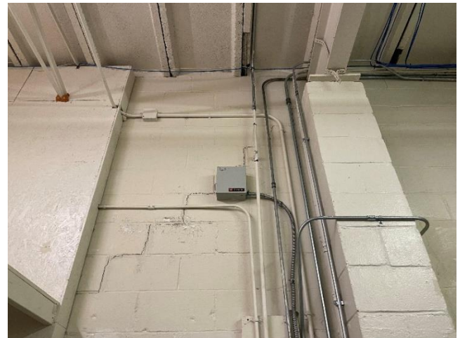
Photo PEB-S1: Spalled Roof Panels and Cracked Masonry Walls
