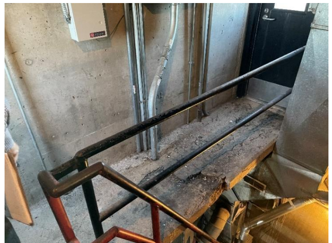
Photo GT8-S1: Deteriorated Walkway Landing
