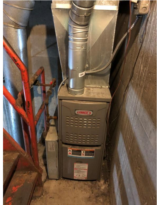
Photo GT8-M1: Existing Gas Furnace
