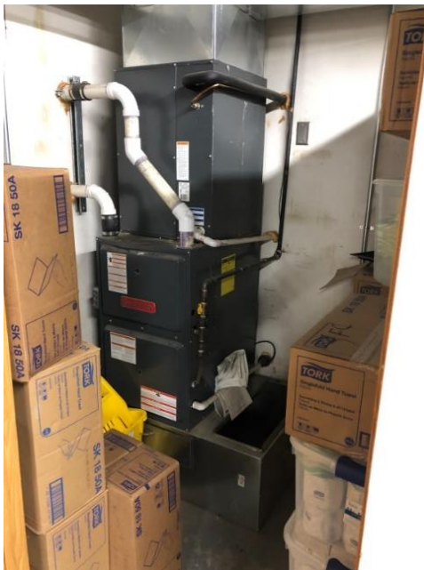
Photo WELL-M2: Typical Existing Gas Furnace
