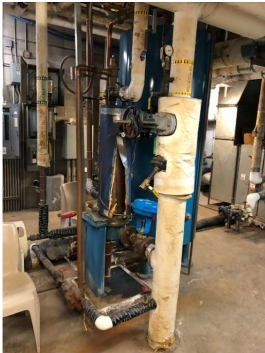
Photo HU7&8-M1: Existing Steam Water Heater
