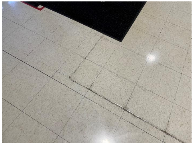
Photo ANC-S2: Cracks in Gym Flooring
