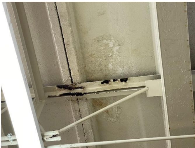
Photo PEB-S2: Rusted Roof Joist
