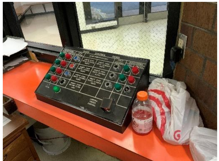
Photo ANC-SEC3: Existing Door Control Panel – Turnkey Entrance
