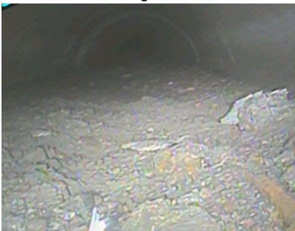
Photo STORM-3: Debris Found in STORM Piping which will Obstruct Water Flow
