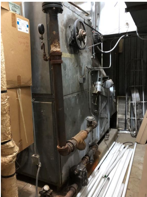
Photo PVB-M2: Existing AHU
