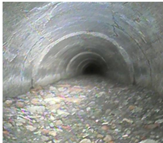
Photo STORM-2: Debris Found in STORM Piping which will Obstruct Water Flow
