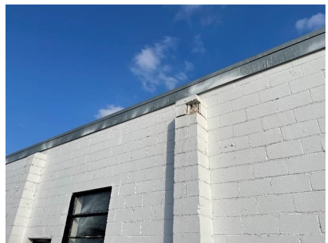
Photo PEB-S3: Spalled CMU at Pilasters
