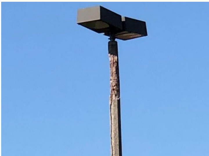
Photo LTG-2: Enlarged Image of Concrete Light Pole South of Housing Unit No. 5. (Note Severe Pole Deterioration with Reinforcing and Interior Conduit Visible)
