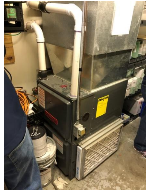
Photo CERT-M2: Existing Gas Furnace Split System
