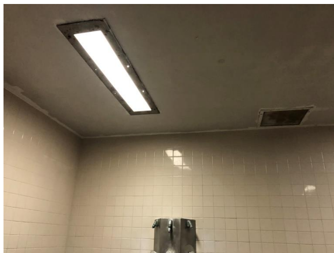
Photo HU7&8-E2: Rusted Lighting Fixture in Shower Area
