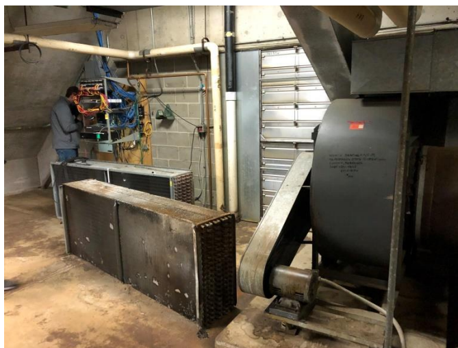
Photo ANC-M4: Changed Out Chilled Water Coils
