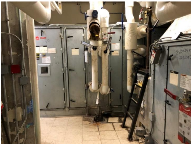
Photo HU6-M6: Typical Existing AHU
