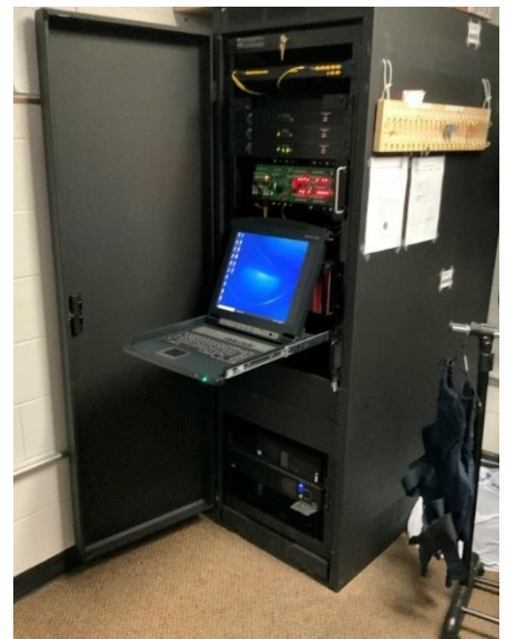
Photo ANC-SEC10: Existing Perimeter Detection System – Head-End Equipment Cabinet (Controller)
