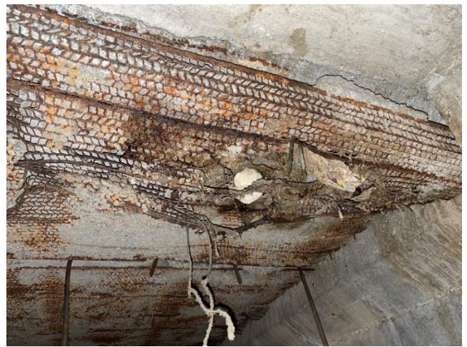
Photo HU6-S2: Damaged Lathe at Steam Tunnel Ceiling
