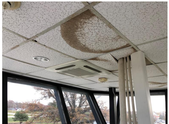
Photo GT1-M2: Existing Ceiling Mounted Fan Coil
