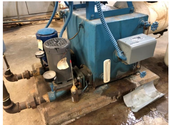
Photo HU7&8-M5: Leaking Steam Condensate Return Pump
