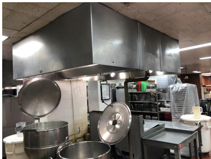
Photo ANC-M5: Existing Kitchen Exhaust Hood
