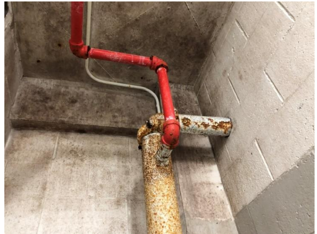
Photo HU6-M4: Rusting and Leaking Fire Sprinkler Piping on Second Floor
