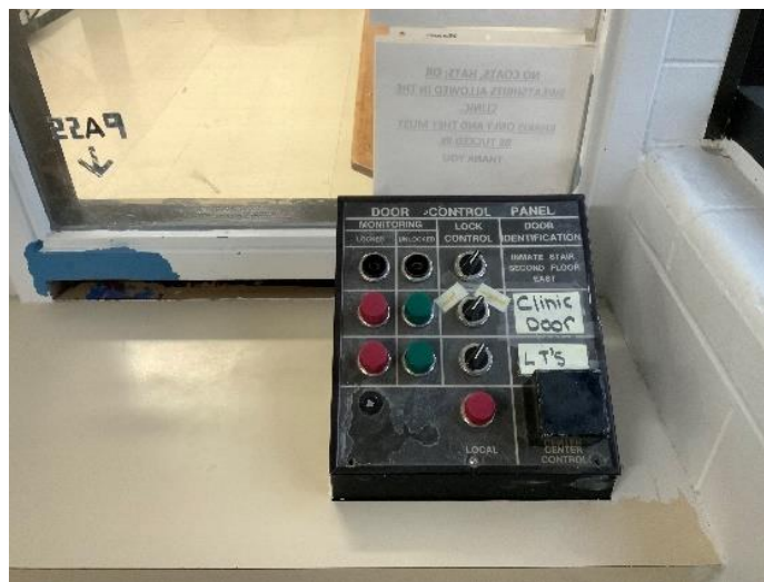
Photo ANC-SEC6: Existing Door Control Panel – Door Control Relays and Switches (behind panels)
