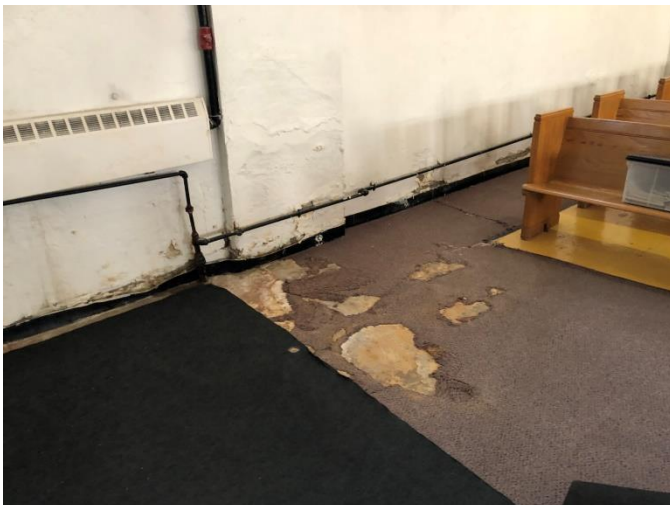
Photo CHAP-M4: Melted/Vaporized Carpet and Rug
