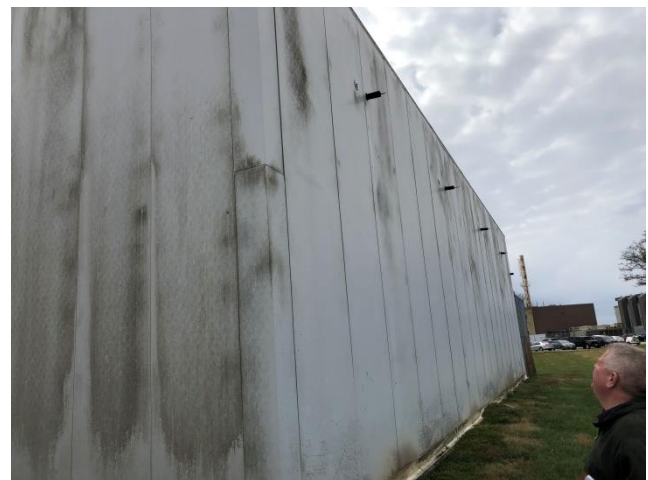
Photo CW-FS6: Existing Evaporator Coil Drains
