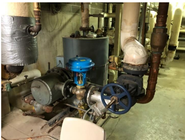
Photo HU6-M1: Existing Steam Water Heater
