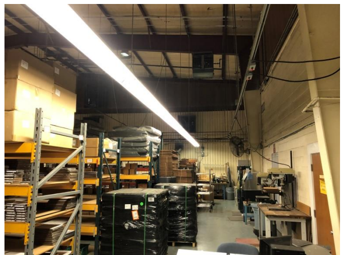
Photo PVB-M1: Gas Piping to Unit Heater
