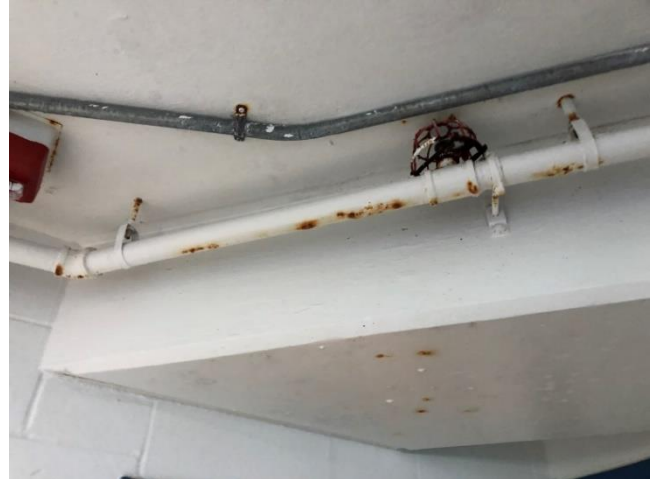
Photo HU1-5-M4: Exposed and Rusting Fire Sprinkler Piping
