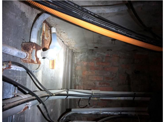
Photo UT-E2: Representative Photo of Rusty Tunnel Lighting. Neither Fixture is Operational
