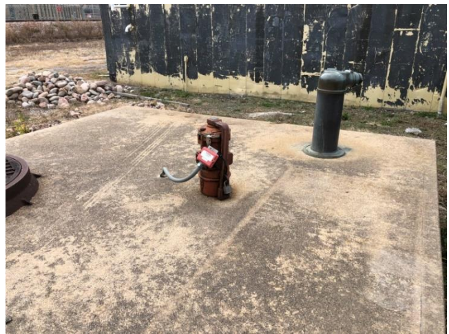
Photo DW&FP-3: Post Indicator Valve Near Central Warehouse
