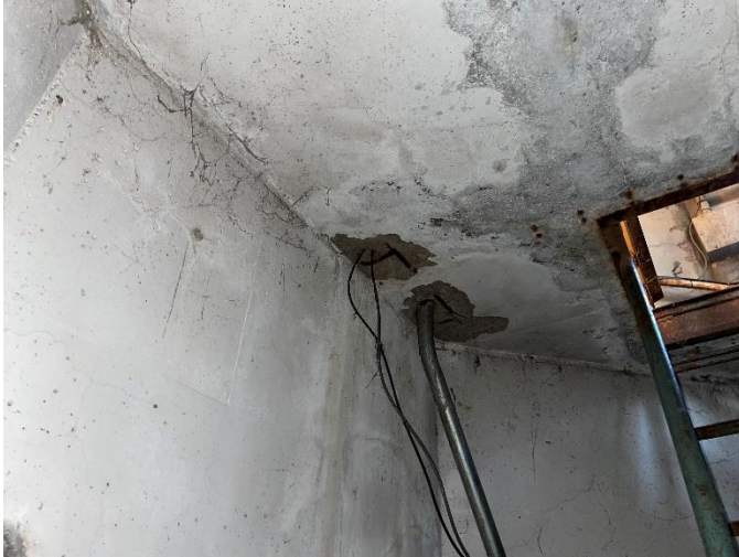
Photo GT5-S1: Spalled Concrete
