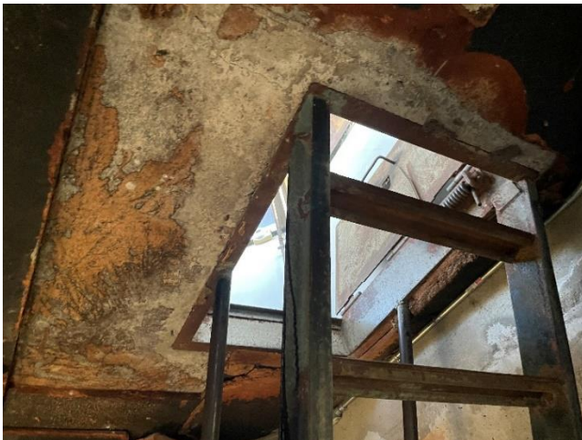
Photo GT6-S4: Deteriorated Concrete at Floor Hatches
