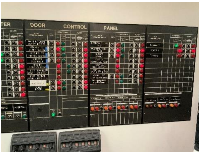
Photo ANC-SEC2: Existing Door Control Panel - Master Control Room
