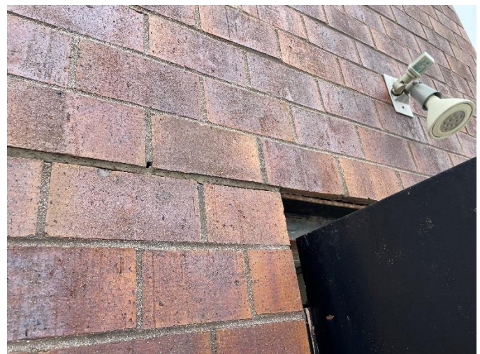
Photo GT1-S1: Failed Sealant
