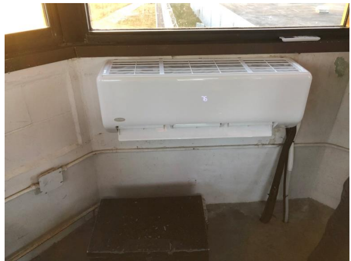
Photo GT5-M1: Existing Wall Mounted Fan Coil
