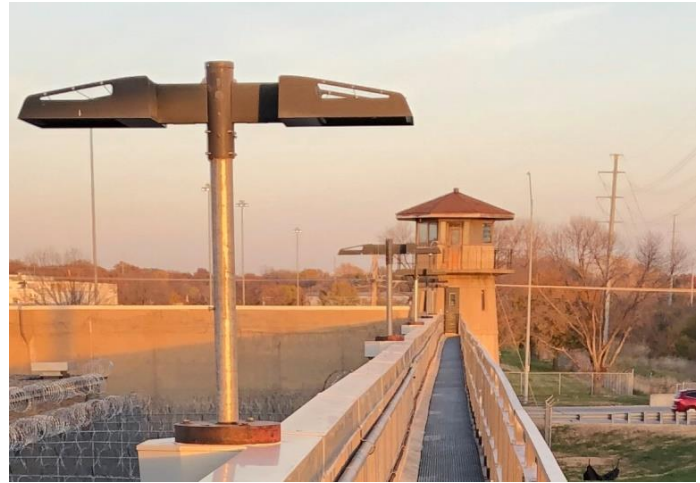
Photo LTG-4: Security Lighting at Wall Between Guard Tower 5 and Guard Tower 6
