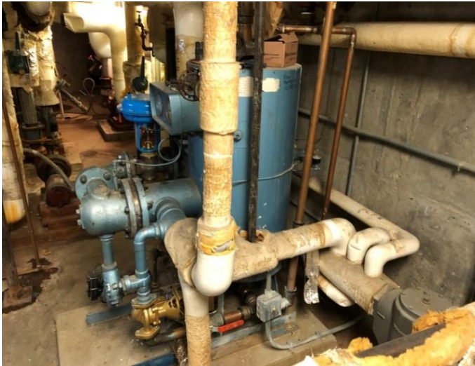
Photo HU1-5-M1: Existing Steam Water Heater
