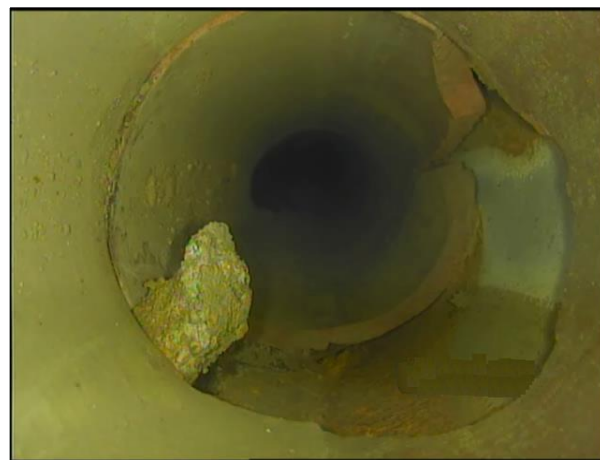
Photo STORM-4: Severely Broken STORM Piping which Needs Immediate Replacement
