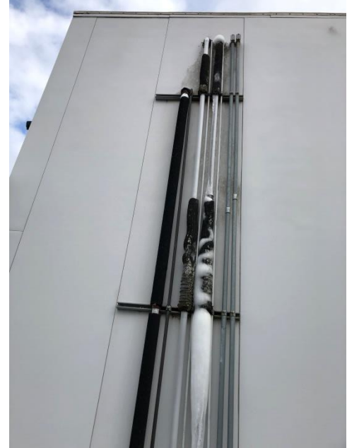
Photo CW-FS4: Existing Refrigeration Piping
