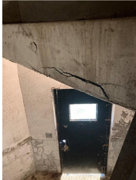
Photo GT6-S3: Spalled Concrete Beam
