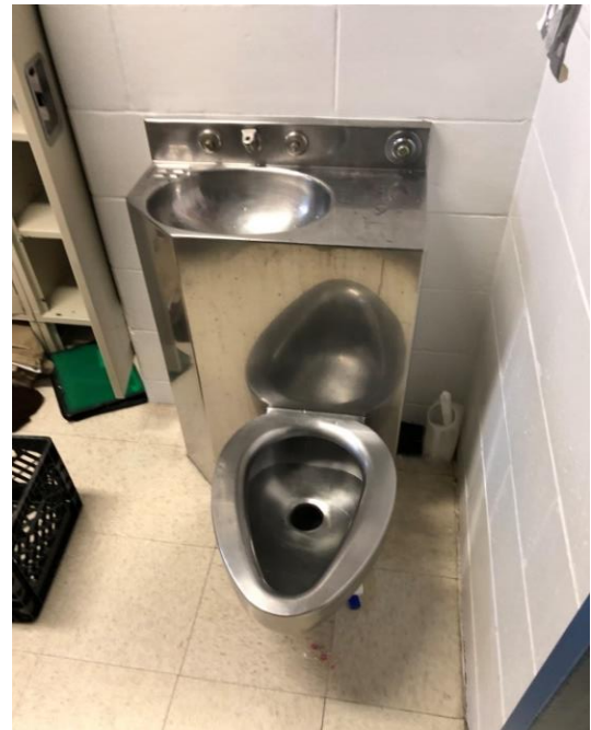
Photo HU1-5-M2: Existing Security Plumbing Fixtures
