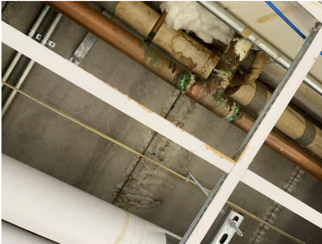
Photo MENT-S1: Water Staining at Roof
