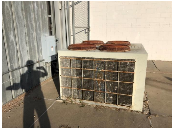
Photo PVB-M3: Existing Abandoned ACCU
