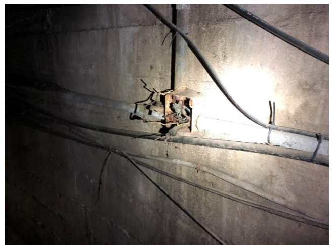
Photo UT-E3: Representative Photo of Rusty Electrical Box with Exposed Conductors
