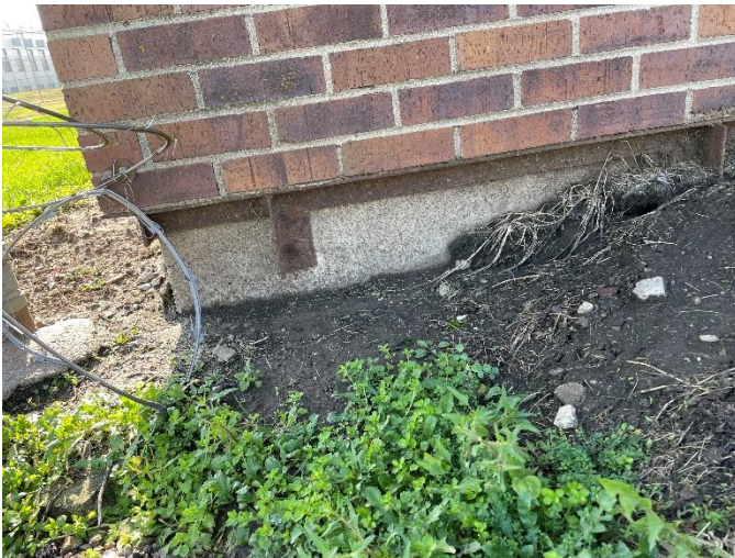
Photo EDU-S1: Brick Wainscot Supported by Steel Angle
