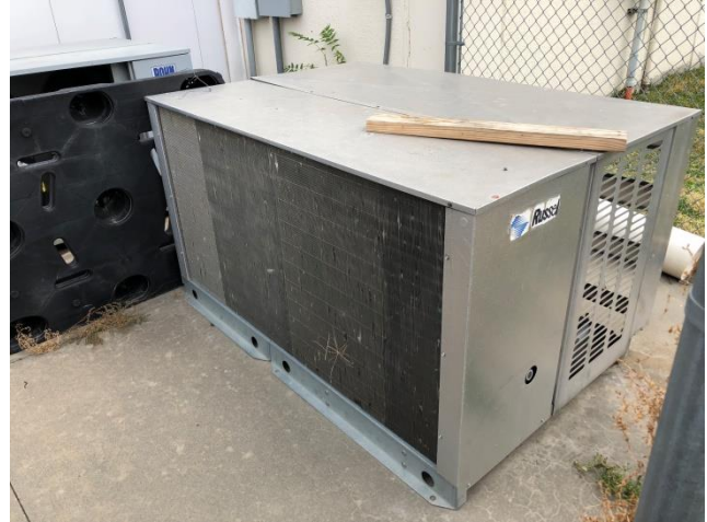
Photo CW-FS8: Existing Large Condensing Unit
