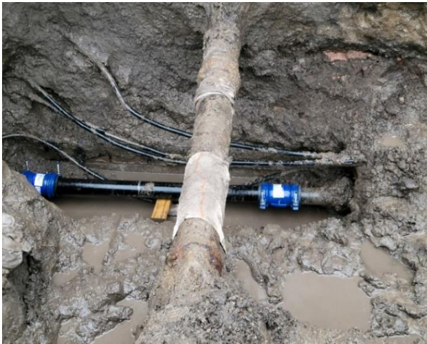
Photo STORM-1: Storm Piping (Top Pipe) Near Housing Unit No. 6
