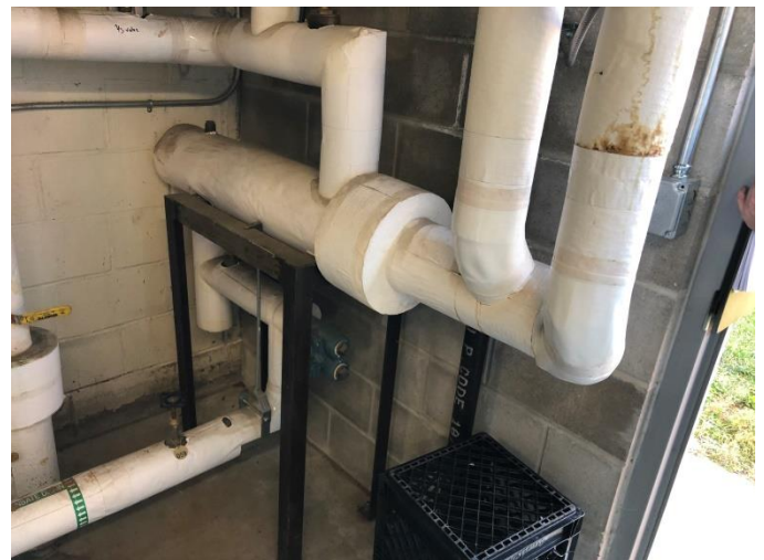
Photo MENT-M1: Existing Steam to Heating Hot Water Shell and Tube Heat Exchanger
