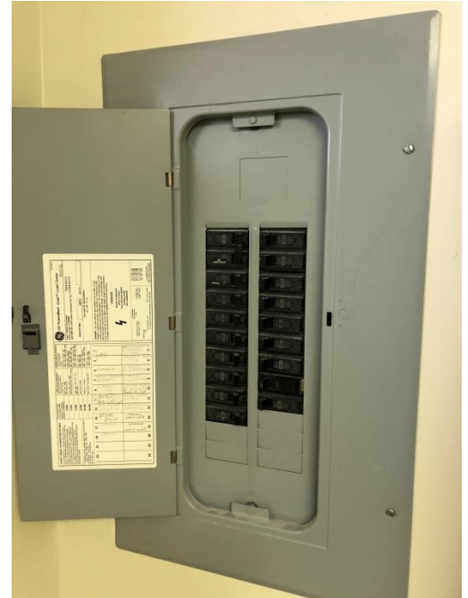
Photo FTO-E1: Main Electrical Panel
