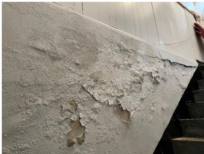
CHAP-S2: Moisture Damage at Tunnel Stair
