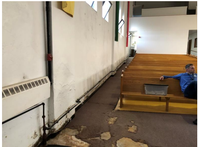
Photo CHAP-M3: Exposed Steam Condensate Piping
