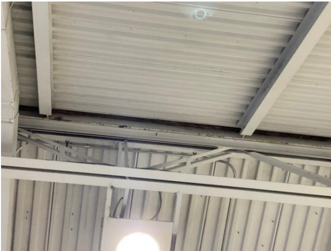
Photo ANC-S1: Rusting Gym Roof Framing
