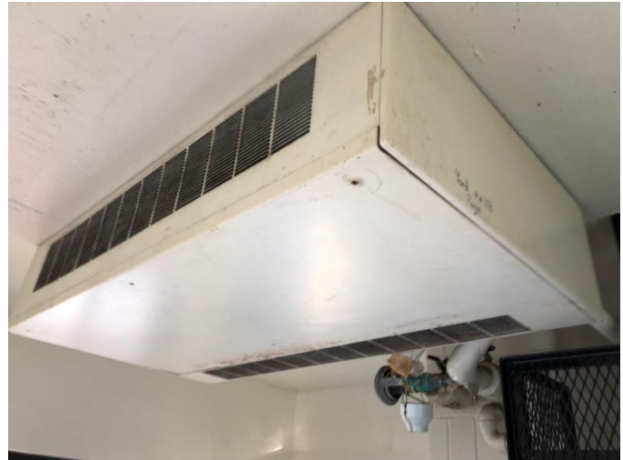
Photo GT10-M1: Existing Ceiling Mounted Fan Coil
