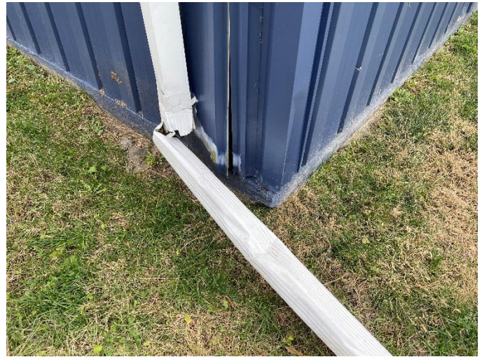
Photo CERT-S2: Example of Impact Damage to Exterior Panels
