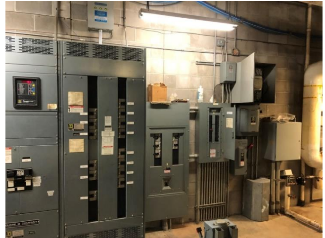
Photo HU7&8-E1: Main Electrical Service
