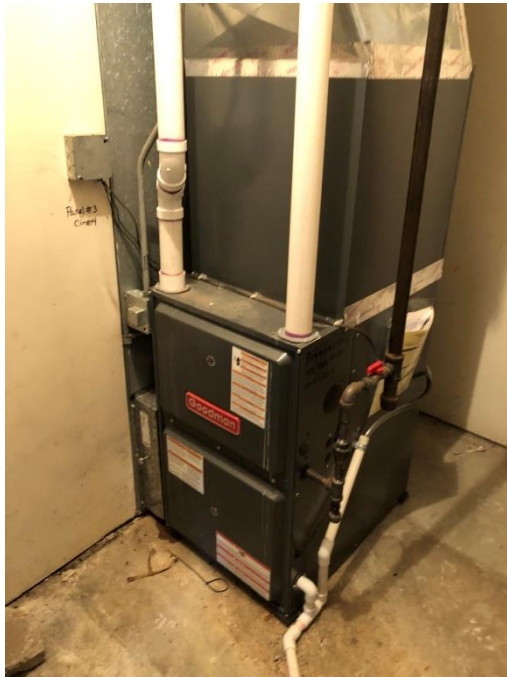
Photo CW-M6: Existing Gas Furnace and ACCU Split System
