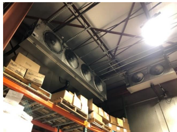
Photo CW-FS2: Existing Freezer Evaporator Coils
