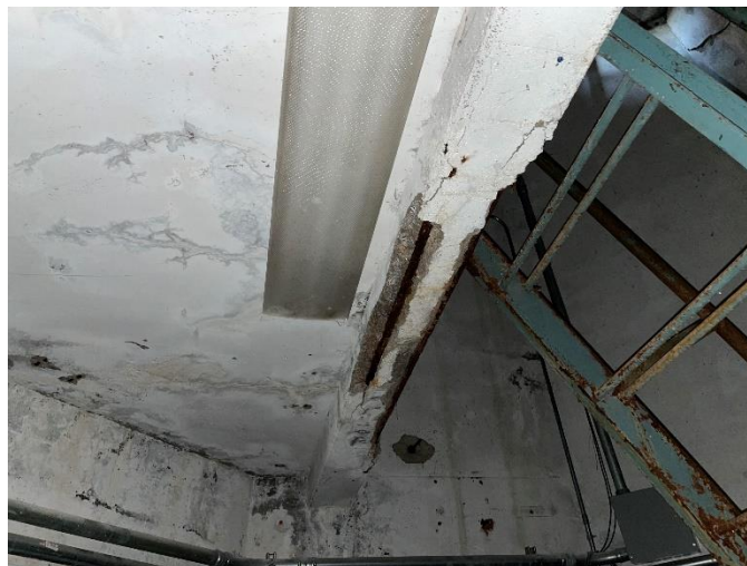
Photo GT5-S3: Spalled Concrete Beam
