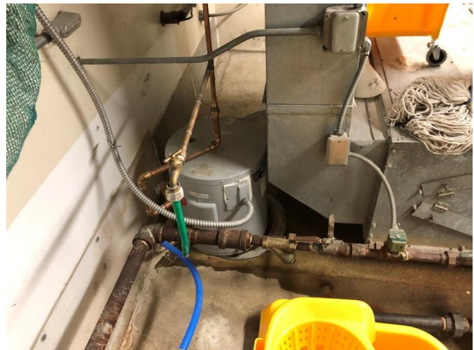
Photo ACT-M1: Existing Electric Water Heater
