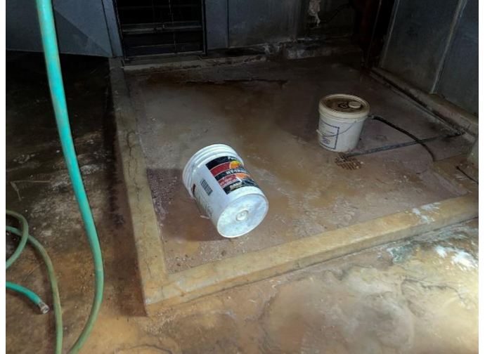
Photo ANC-S4: Deteriorated Curb in Mech Room 2B68 Foodservice
