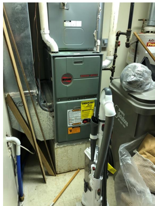
Photo FTO-M2: Existing Gas Furnace Split System
