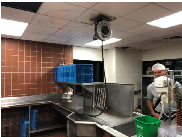
Photo ANC-FS18: Existing Hose Reel Spray Assembly
