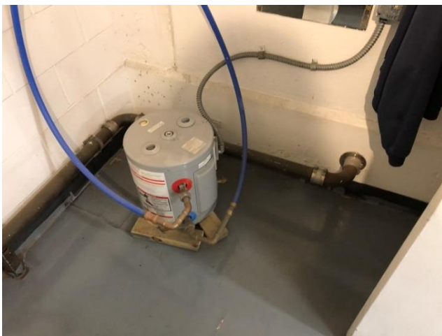
Photo CW-M1: Typical Existing Electric Water Heater
