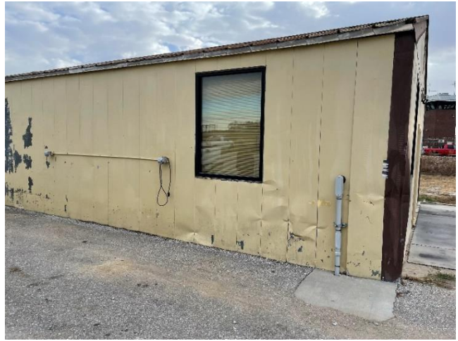
Photo WELL-S2: Damaged West Wall
