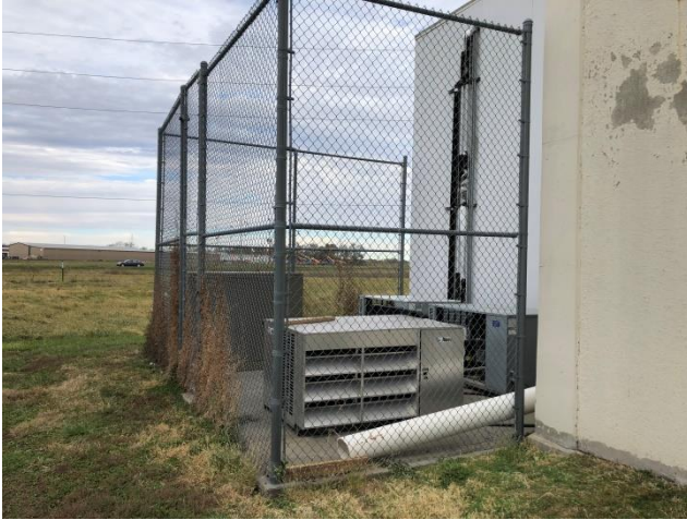
Photo CW-FS7: Existing Freezer Condensing Units
