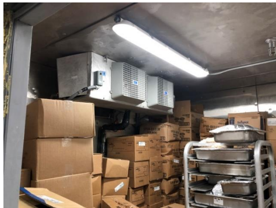
Photo HU6-FS4: Existing Freezer Evaporator Coil
