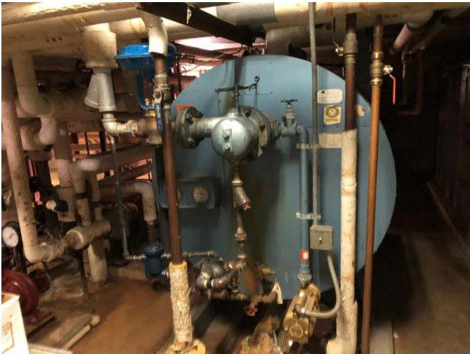
Photo ANC-M1: Existing Steam Water Heater
