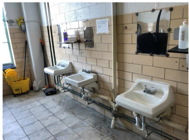
Photo HU6-M2: Exposed Restroom Plumbing
