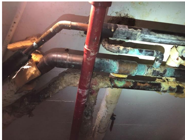
Photo HU6-M5: Rusting Fire Sprinkler Piping on First Floor
