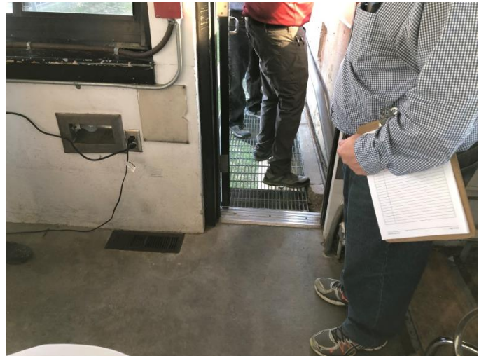
Photo GT7-M1: Existing Floor Mounted Supply Air Register
