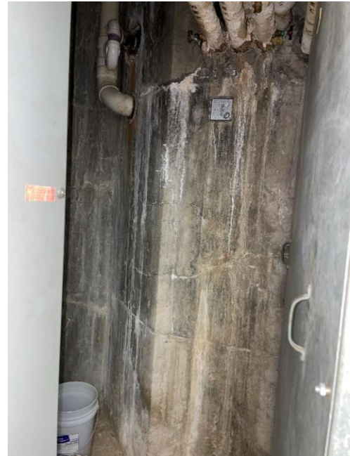
Photo HU1-5-S1: Cracks in Mechanical Room Wall
