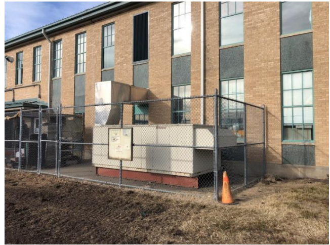
Photo HU6-M7: Existing Kitchen Make-Up Air Unit
