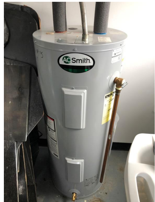
Photo CERT-M1: Existing Electric Water Heater
