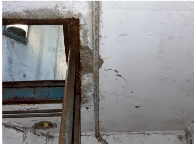
Photo GT6-S4: Deteriorated Concrete at Floor Hatches
