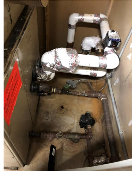
Photo EDU-M2: Piping Connections to AHU
