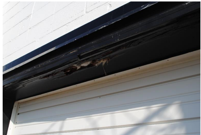
Photo PEB-A1: Overhead Door Damage at Pre-Employment Building.
