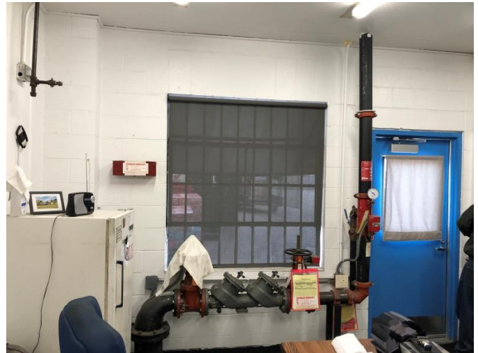
Photo CW-M3: Fire Protection Water Service Entrance
