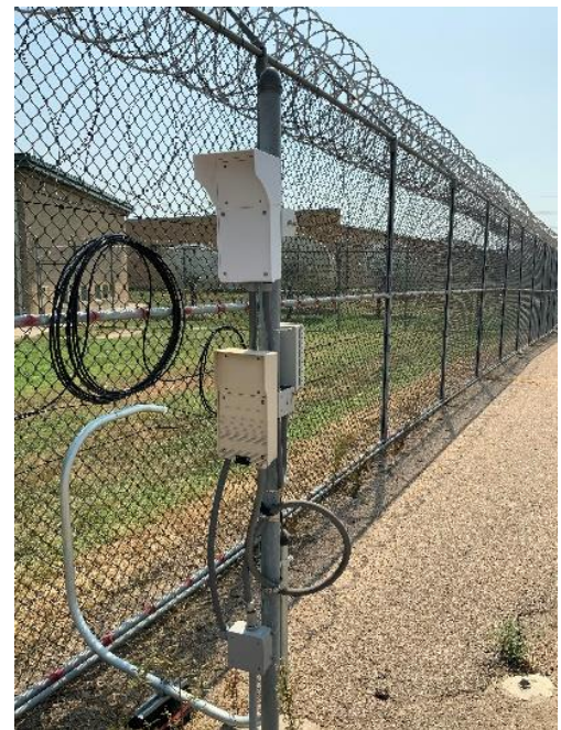
Photo S-SEC-2: Microwave Transmitters – Part of the Senstar Fiber Patrol System PDS
