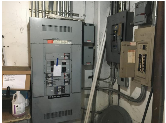
Photo CW-E1: Main Electrical Service
