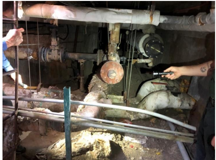
Photo CWS-1: Chilled Water Piping (Left to Right, Down Low) in Tunnel NE of Laundry
