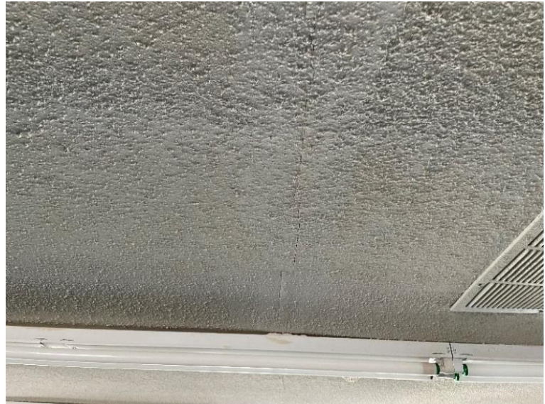
Photo LIB-S1: Cracked Gypsum Sheathing
