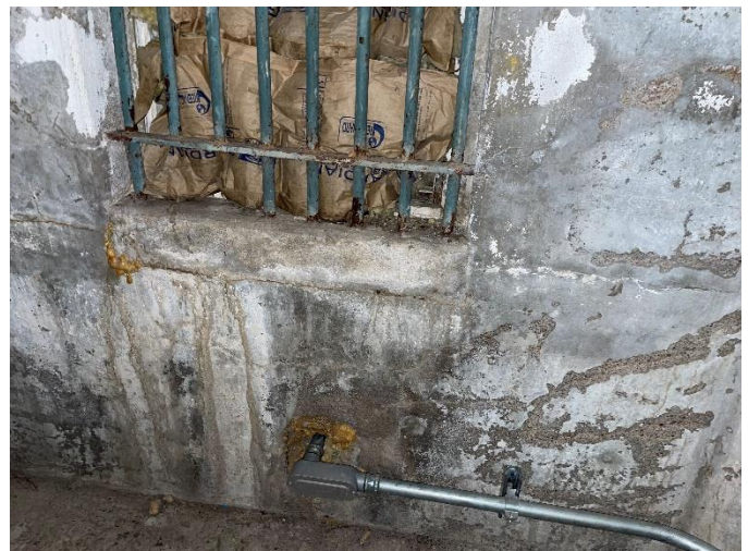
Photo GT4-S3: Concrete Deterioration at Window
