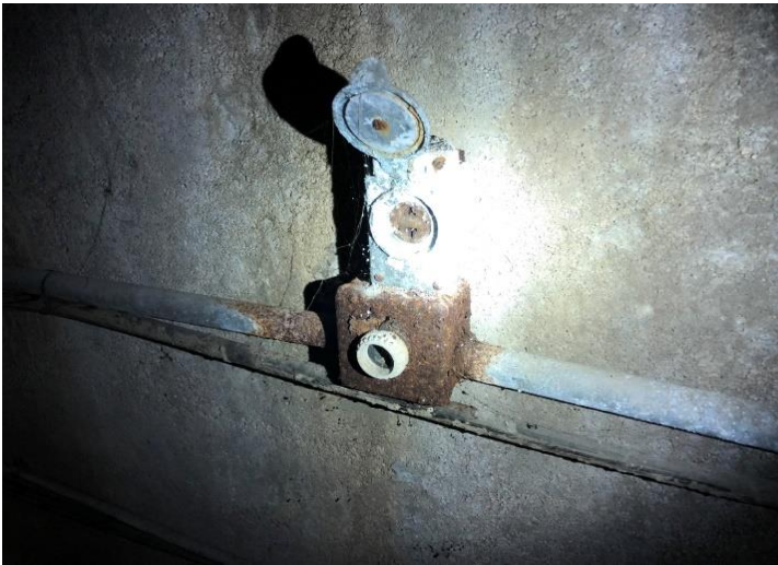
Photo UT-E1: Representative Photo of Rusty Tunnel Lighting and Receptacle Box, Lamp is Missing
