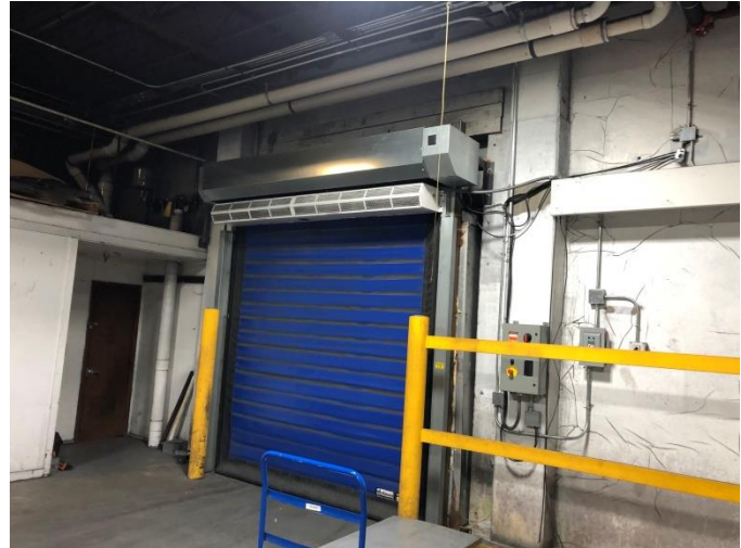
Photo CW-M7: Existing Air Curtain at Rapid Open Freezer Door
