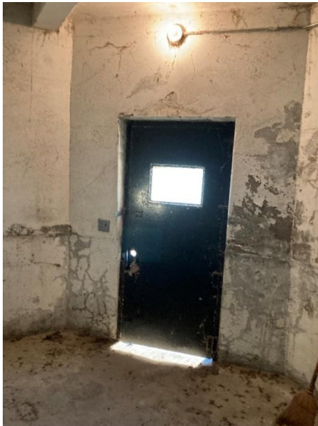
Photo GT6-S2: Map Cracking in Walls
