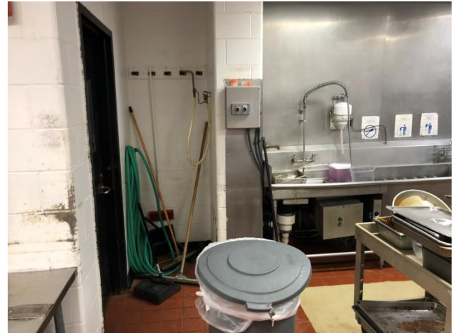
Photo ANC-FS17: Existing Pre-Rinse Assembly
