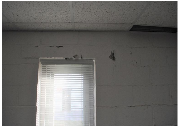
Photo MENT-A1: Interior Wall Damage Above Window
