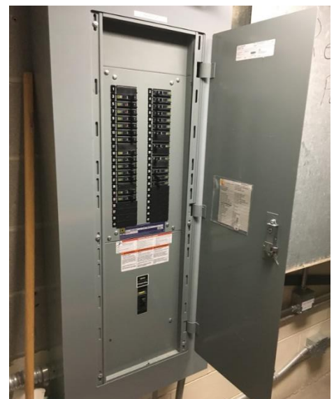
Photo GT3-E1: Existing Electrical Panel
