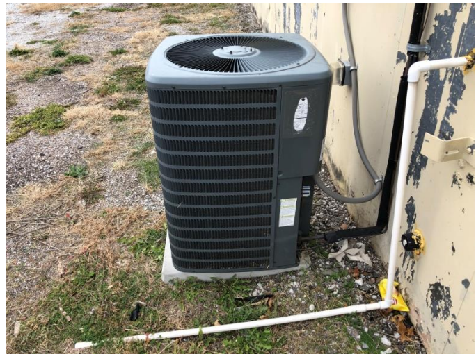
Photo WELL-M3: Typical Existing ACCU
