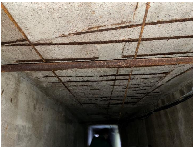
Photo UT-S1: Deteriorated Tunnel Lid
