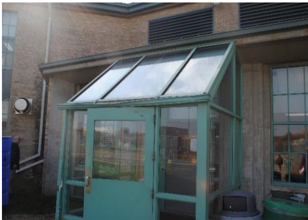
Photo HU6-A1: Weather Vestibule with Worn Door Hardware and Damaged Window Framing
