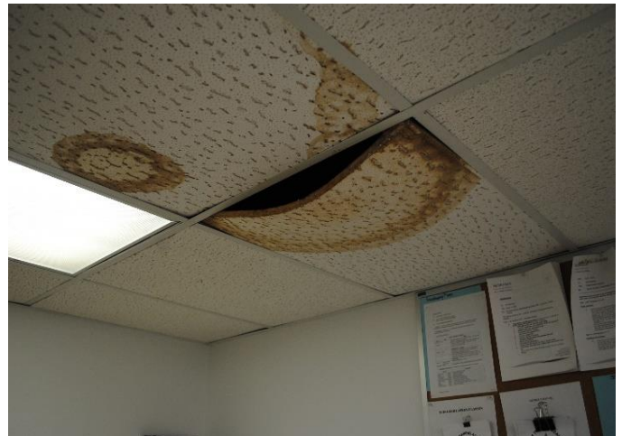
Photo FTO-A1: Typical Ceiling Stain
