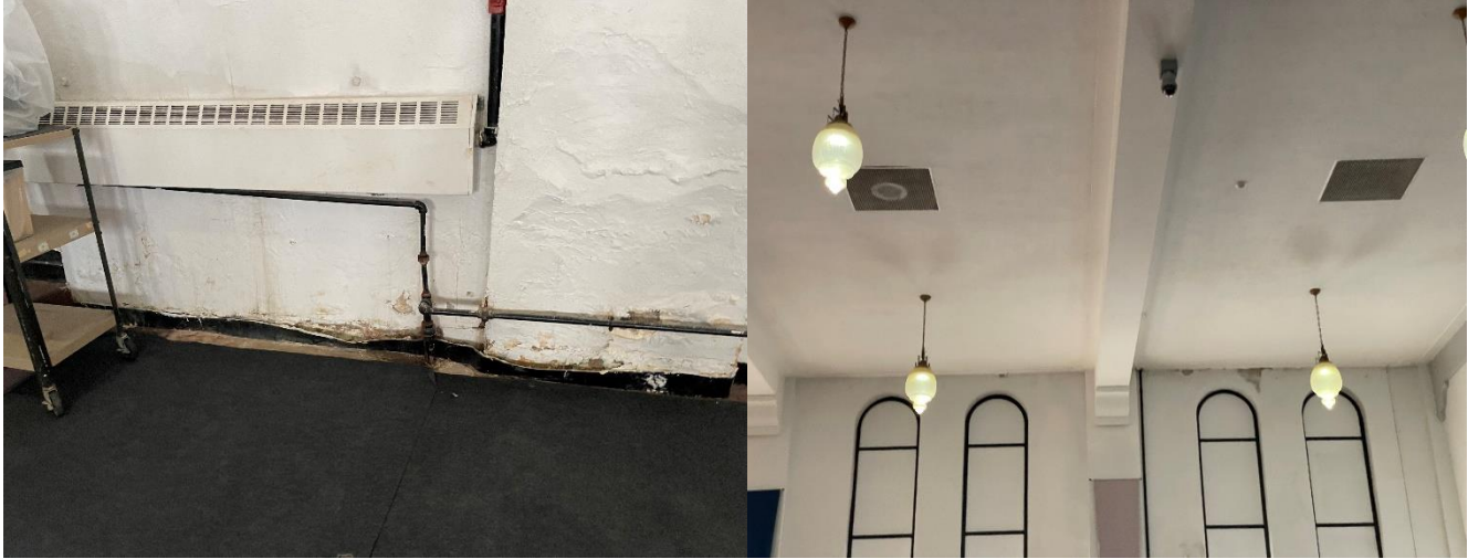
CHAP-S1: Moisture Damage at Lower and Upper Wall
