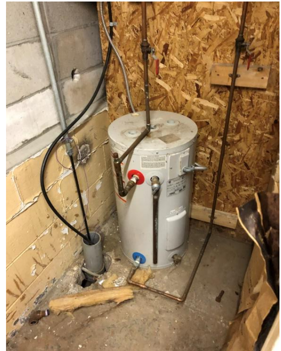
Photo PEB-M1: Existing Electric Water Heater
