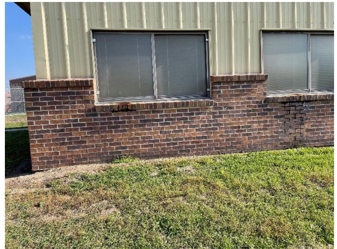
Photo EDU-S2: Sealant and Moisture Issues
