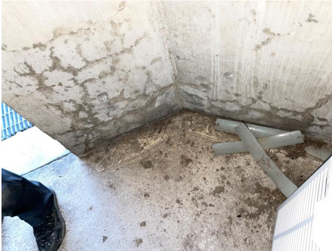
Photo GT4-S2: Map Cracking
