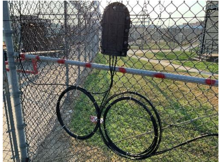
Photo S-SEC-1: Fence Mounted Fiber Sensor Cable – Senstar Fiber Patrol System
