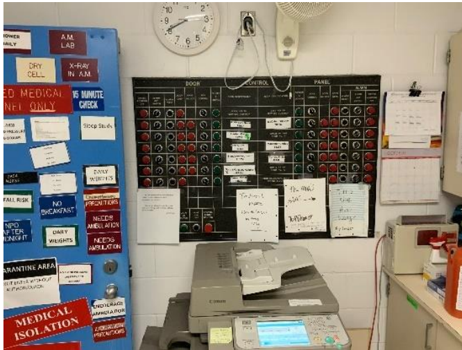
Photo ANC-SEC4: Existing Door Control Panel – Nurses Office
