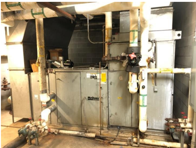
Photo HU7&8-M4: Typical Existing AHU
