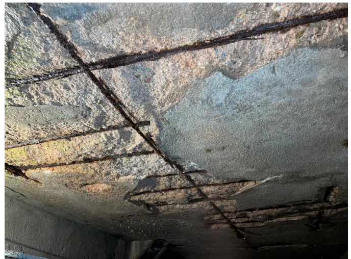
CHAP-S3: Deteriorated Tunnel Lid
