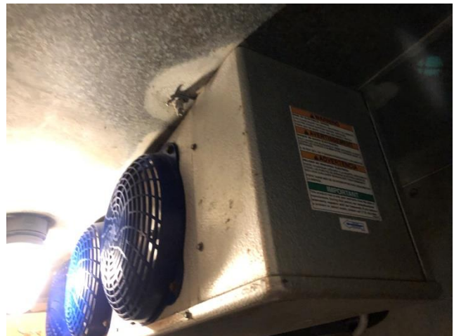
Photo ANC-FS23: Existing Walk-in Evaporator Coil
