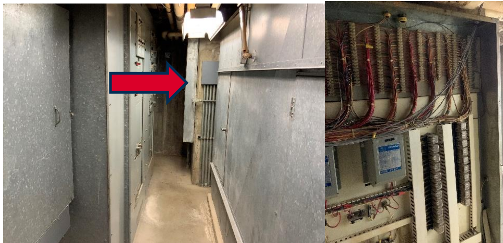
Photo HU1-SEC3: Existing Door Control Enclosures-Typical for both A and B Wing
