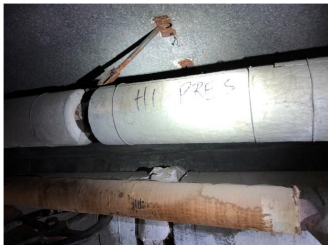
Photo STM-2: Bent Steam Pipe Hanger in Tunnel West of Chapel
