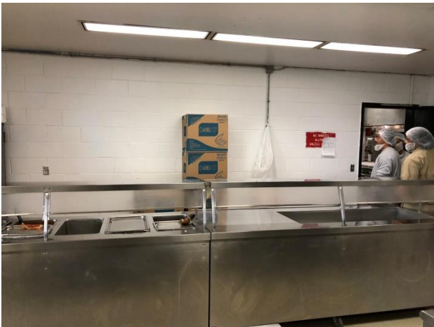
Photo ANC-FS12: Existing Refrigerated Counter
