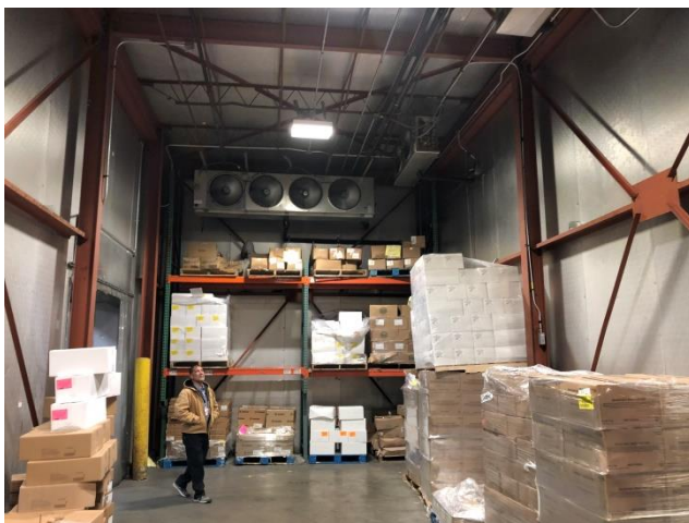
Photo CW-FS5: Existing Freezer Evaporator Coils
