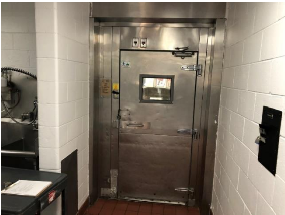
Photo HU6-FS1: Existing Walk-in Cooler Door
