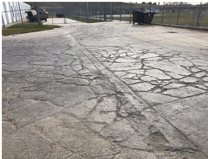
Photo PAVE-1: Poor Pavement Near HU6
