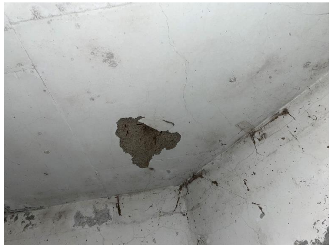
Photo GT4-S1: Spalled Slab
