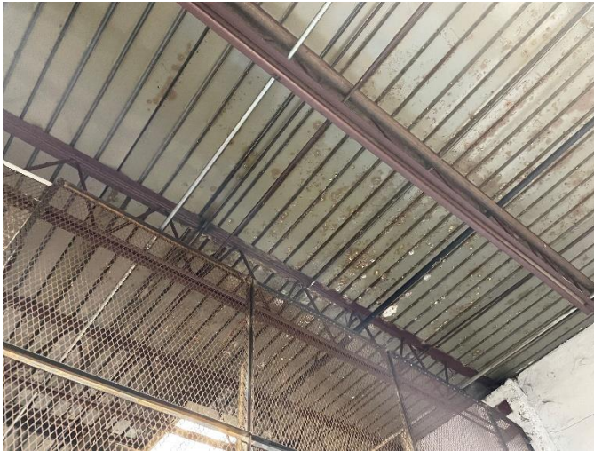
CW-S2: Rusted Roof Deck Installed Upside Down
