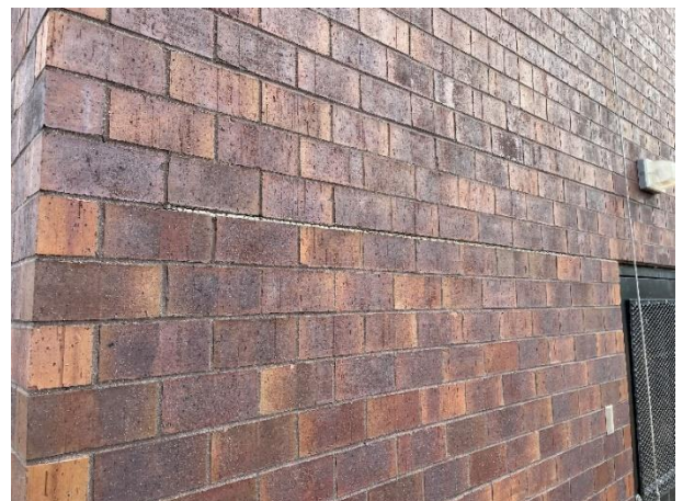
Photo GT3-S1: Failed Sealant
