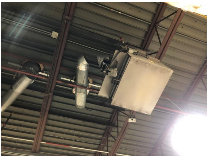
Photo CW-M4: Existing Abandoned Gas Unit Heater
