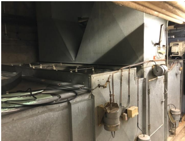
Photo HU1-5-M7: Existing Pneumatic Controls
